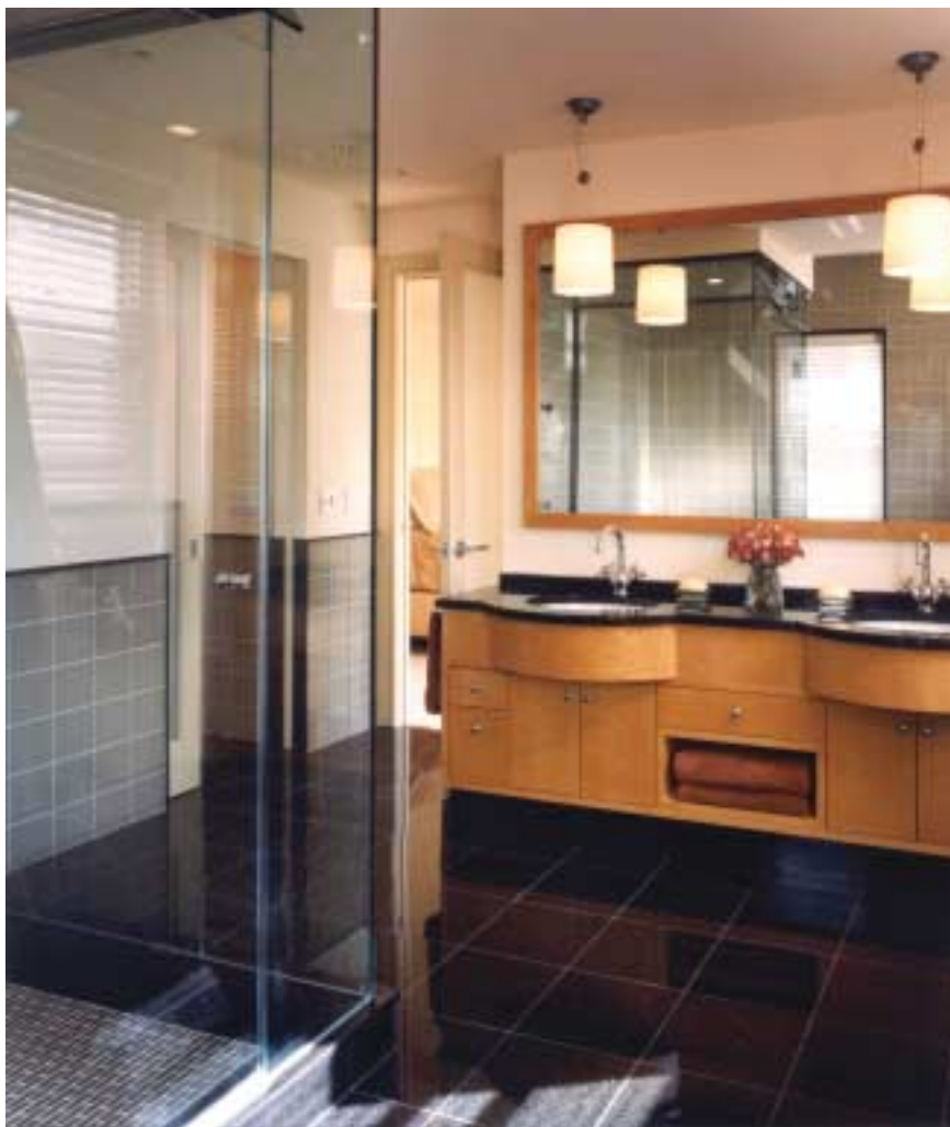
The bathroom floor of the residence features 12- x 12-inch tiles of Black Galaxy granite, and a 1¼-inch-thick slab of the same granite was used for the vanity top.
