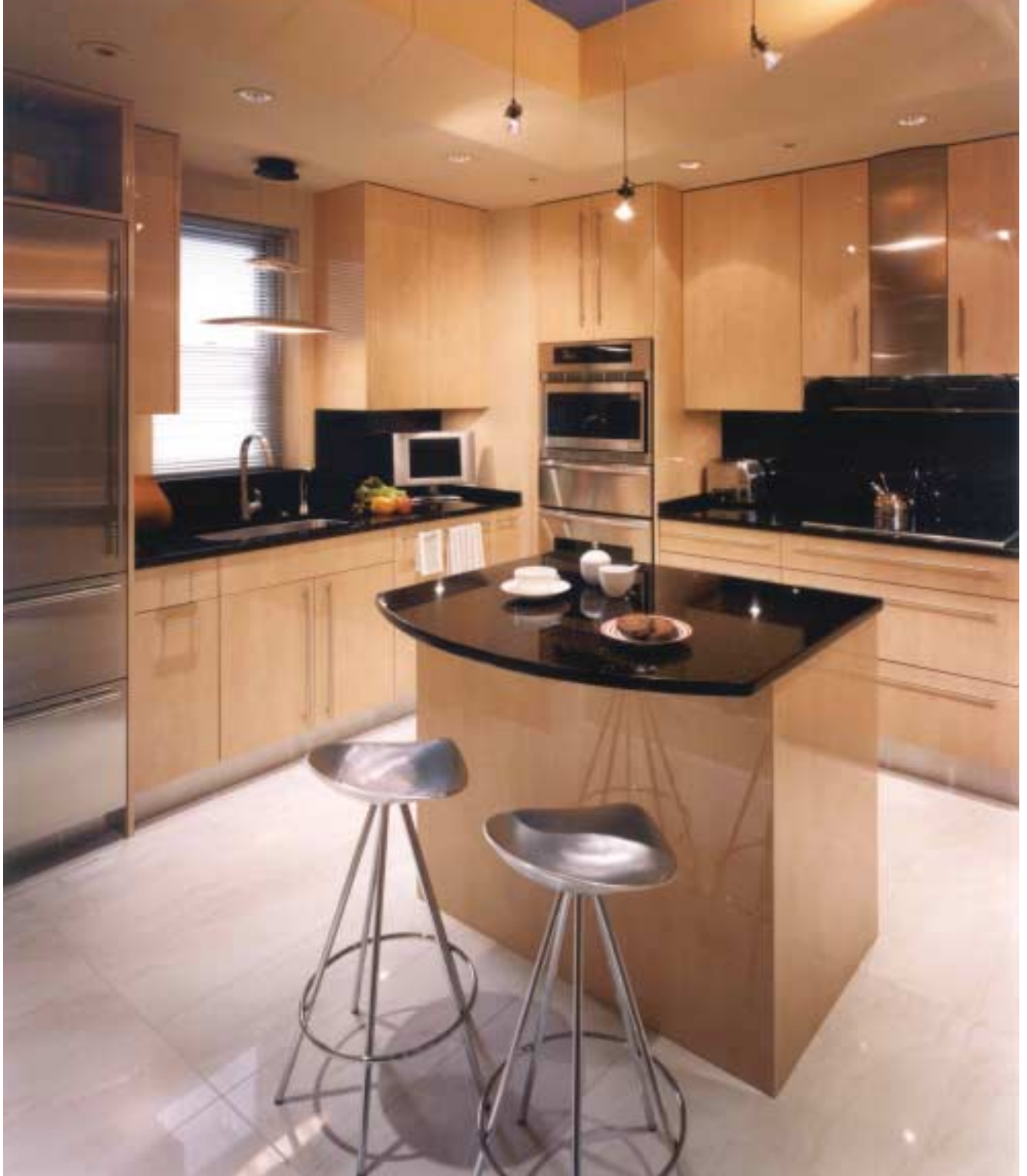
In the kitchen of the Rittenhouse Square home, the countertops were fabricated from 1¼-inch-thick slabs of Black Galaxy granite, and the floor is comprised of Graniti Fiandre 2- x 2-inch and 2- x 16-inch tiles.
